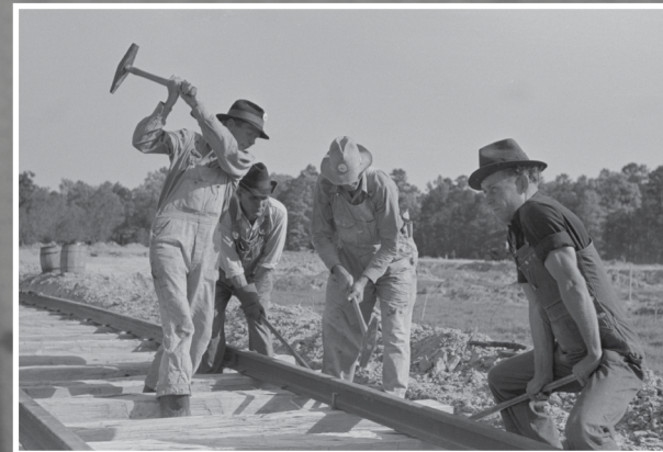
Railroad gang, Southern Paper Mill construction crew. Lufkin, Texas. Russell Lee. April 1939.
